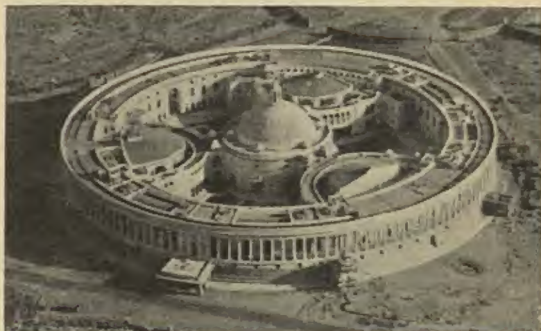
COUNCIL AND ASSEMBLY BUILDING, DELHI
